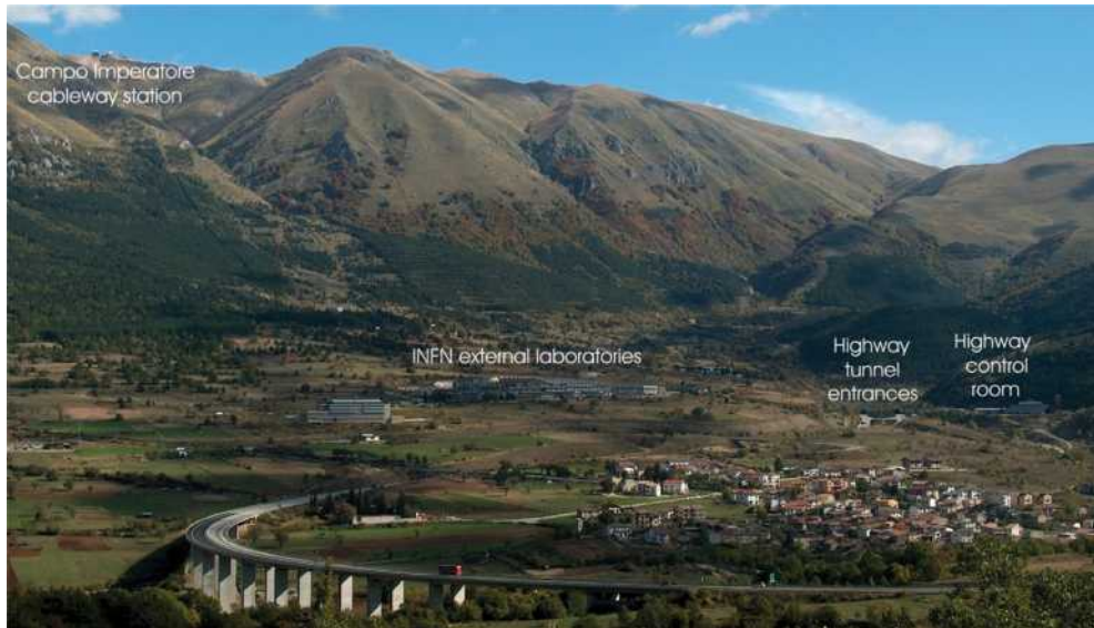
Figure 1: Partial view of Gran Sasso Mountain from L'Aquila side.
