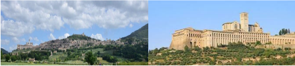
Figure 1: (a) Panoramic view of Assisi where the Sacred Convent is visible on the left; (b) Panoramic view of the Papal Basilica and the Sacred Convent of Saint Francis in Assisi.
